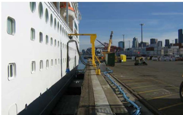
Fig. 15. Shore Power Connection (Terminal 30) (Note: Blue hose - potable water utility connection.)
